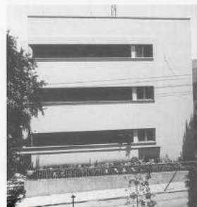
29 Idelson st. - 1936, Architect: Dov Karmi Recessed Balconies provide a local equivalent to Corbusian ribbon windows
