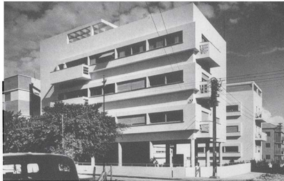
Engel House - 1934, Architect: Zeev Rechter, A vision of the city on pilots, influenced by Le Corbusier
